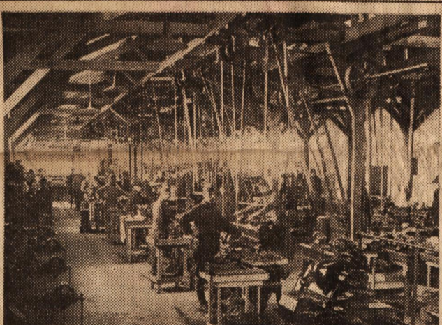
SOUTH END OF MACHINE SHOP
